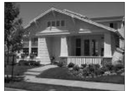
ABOVE: Desirable These examples of infill houses in traditional neighborhoods utilize site plans and architectural designs that reflect the street orientation and scale familiar to the street.
